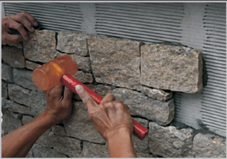
Fixing the cladding
