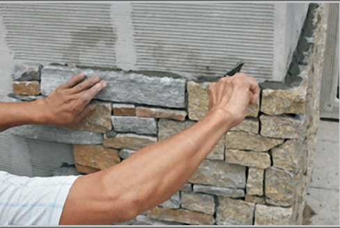
Attaching and aligning the cladding to the kitchen module
