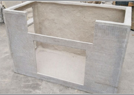
Making cut-out for built-in grill and doors
