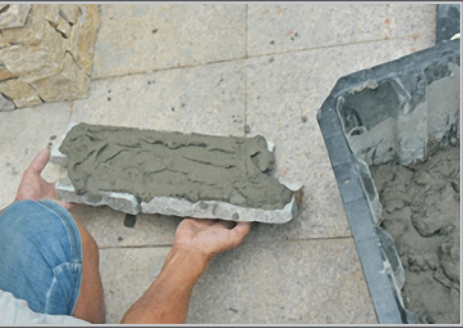
Apply suitable adhesive to the cladding
